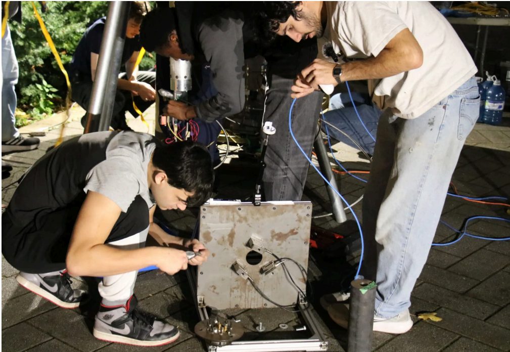
Fig. 3.2: Electrical and control system wiring integration for the test stand.
